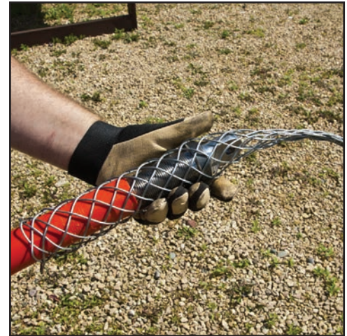
Figure 29. Installing Pulling Grip
