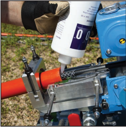
Figure 54. Add Lubricant Behind Cable Assembly
