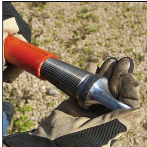
Figure 7. Installing Conduit Pulling Eye
