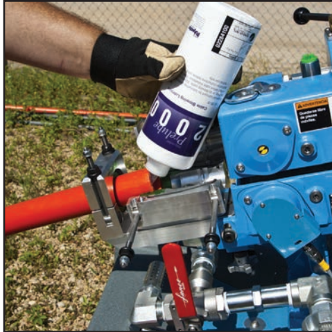
Figure 52. Add Lubricant before Cable Assembly
