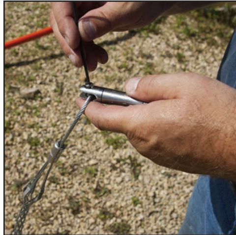
Figure 47. Install Swivel on Cable Grip
